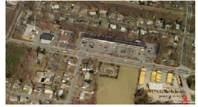
Rt. 25A between Tesla St. and Miller Ave.
