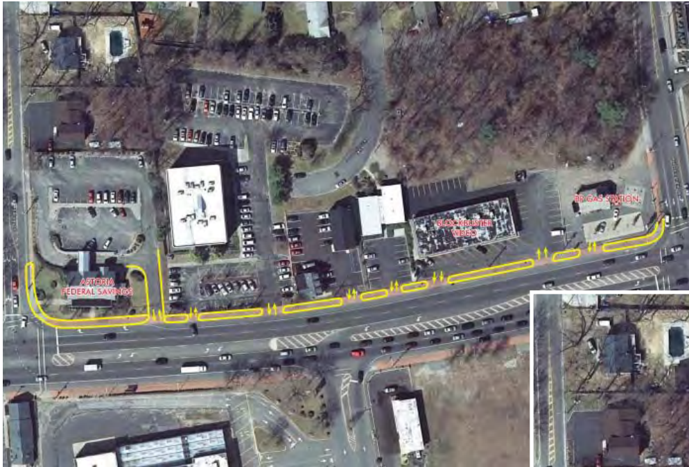
Before Access Management
