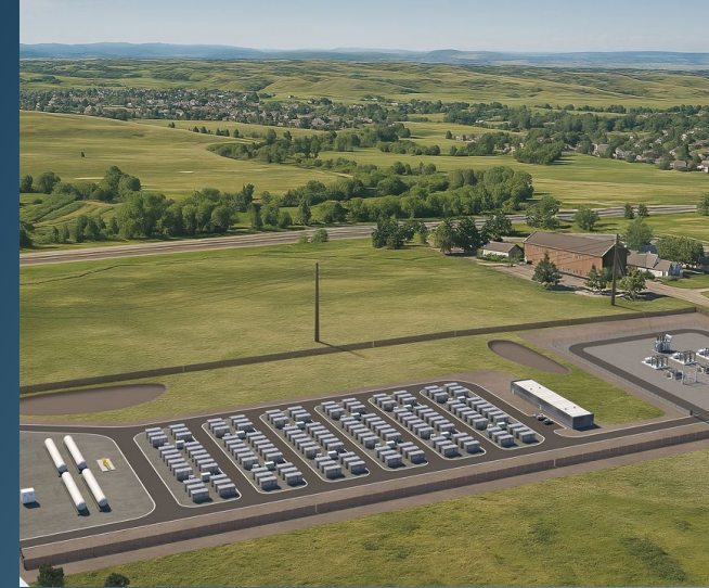
36 Mw of Linear Generators for an Electric Cooperative in Colorado
